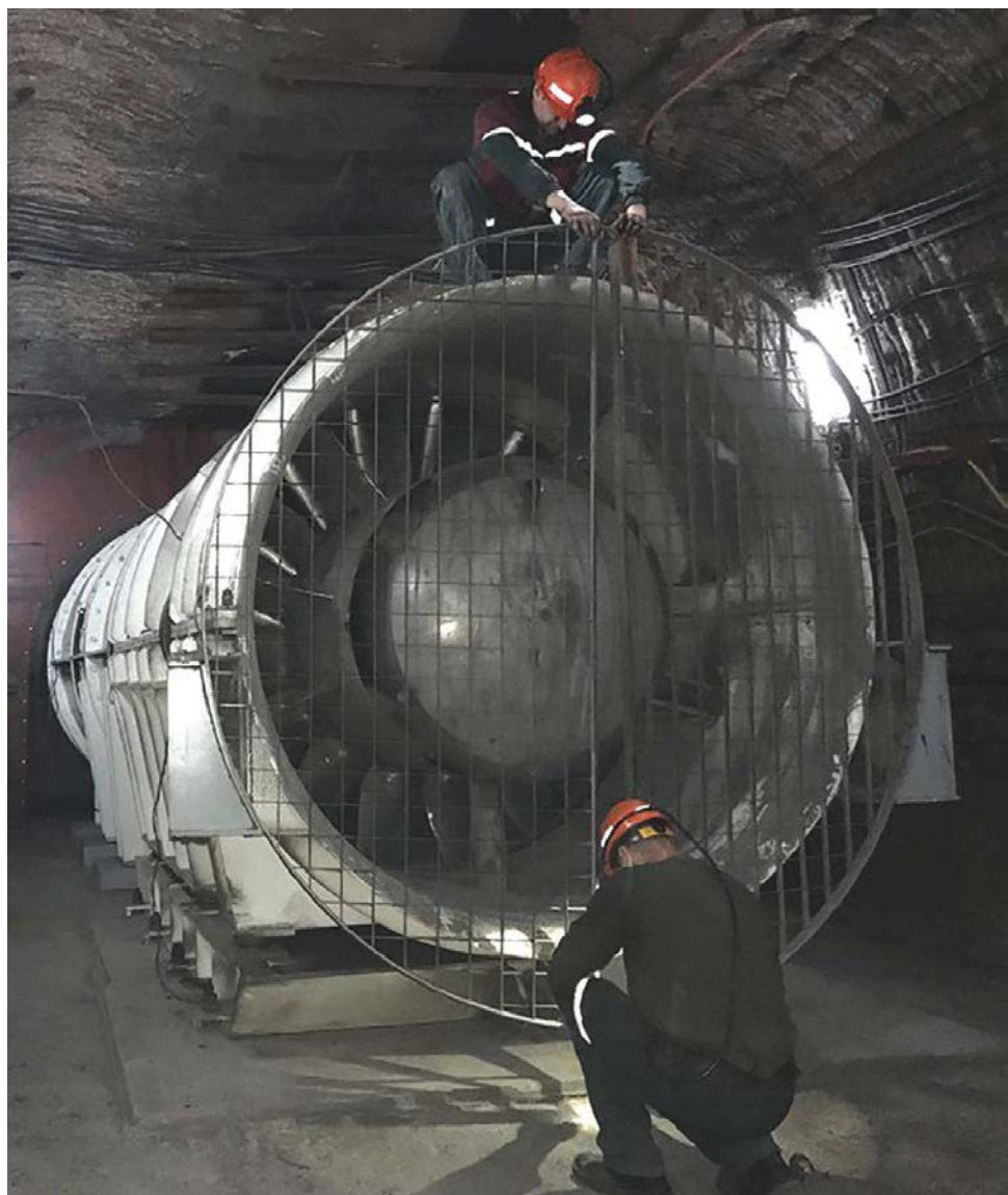
Above, CFE engineers install fans and attenuation systems. (Photo: LMS)
