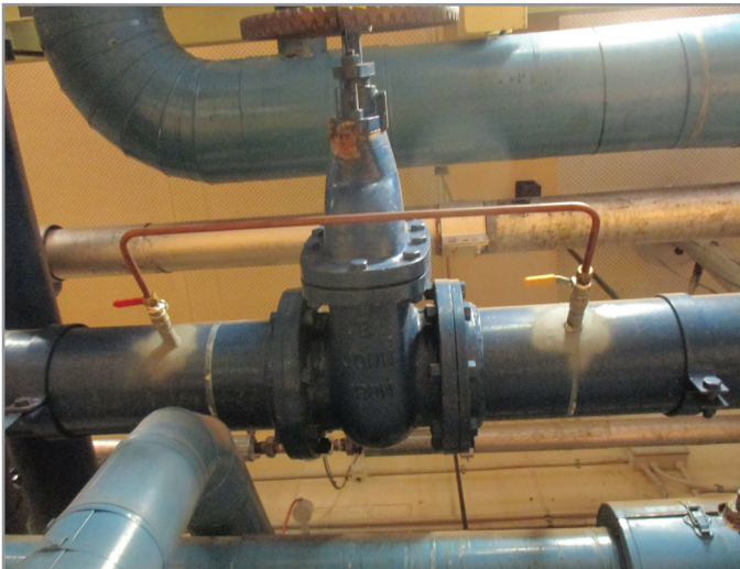
Figure 5.1-2: Solution for managing dead legs (small-bore bypass)
