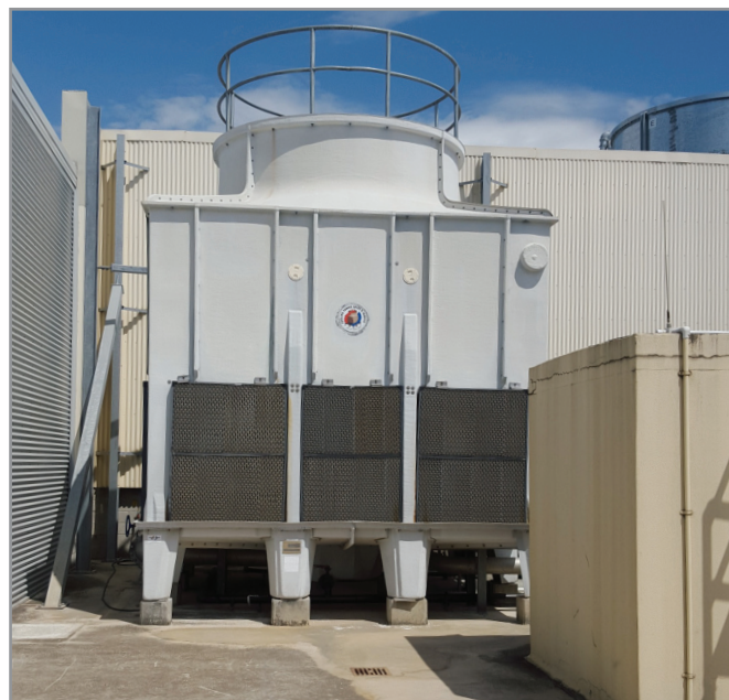
Figure 5.5-2: A cooling tower with no walkway or platform to allow removal of access panels for inspection and maintenance
