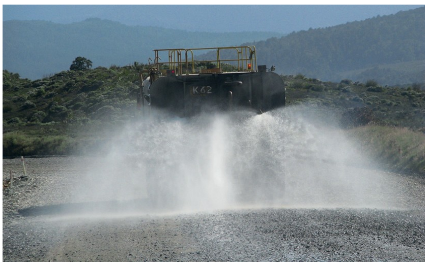
Figure 4: Dust suppression using a mobile tanker.
