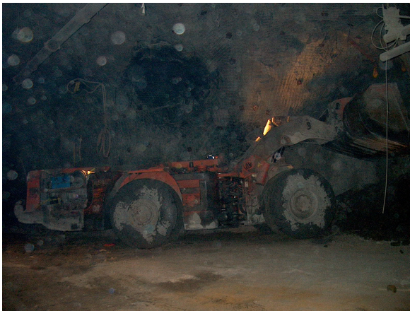
Figure 11: LHD in operation dumping ore on 8000 Level (-7000ft).
