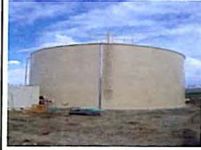
Million gallon tanks
