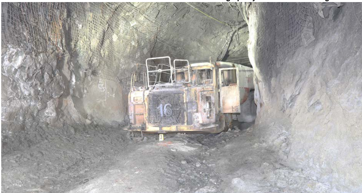
Photo 1: Burned out truck in metalliferous mine decline. Photograph by NSW Resources Regulator.
