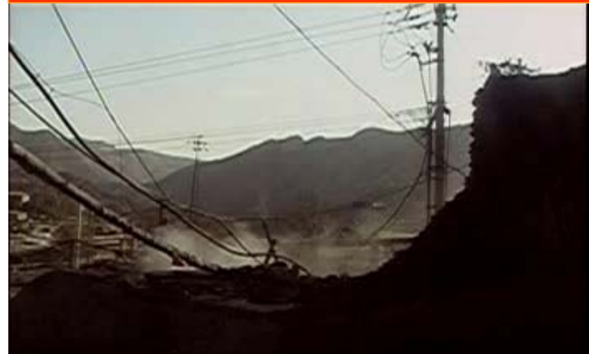
The destruction of ventilation equipment room
