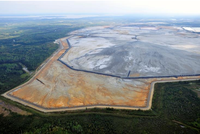
Loss of Containment of Water Treatment and Tailings Ponds
