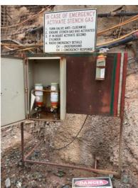
Left. Stench gas activation station (yellow circle) located within 50 metres of a portal, mounted on combustible material and adjacent to a potential ignition source. Right. Stench gas bottles installed to manufacturer's specifications with activation instructions provided.
