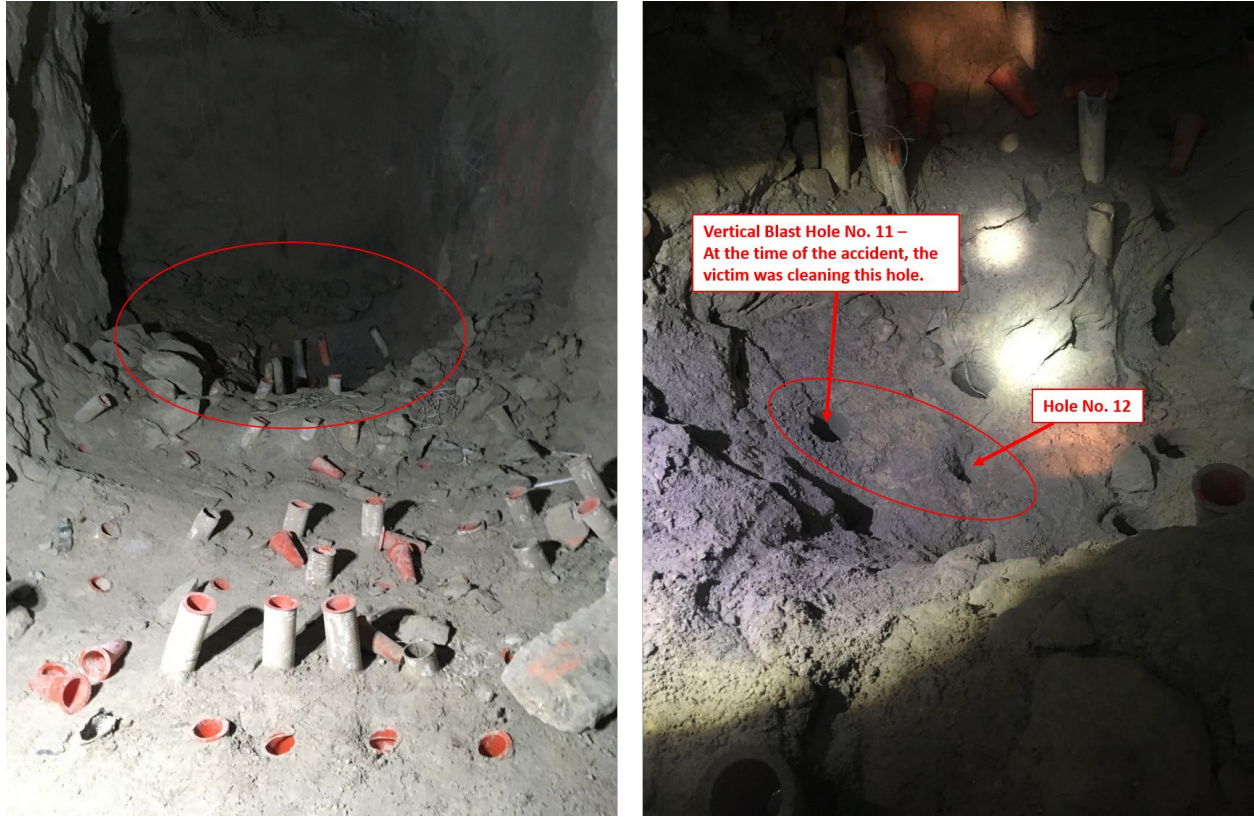
Figure 3 - MP2730 Level - Stope 2805 Development Area - Accident Scene
