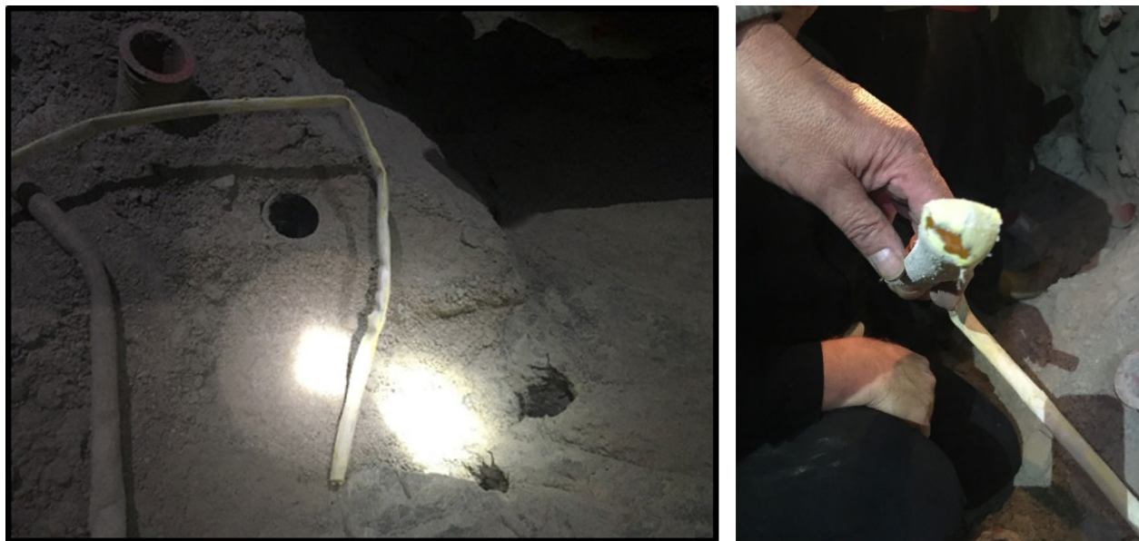
Figure 4 - Photos of Grout Line Used by the Victim (Note: Damaged End)
