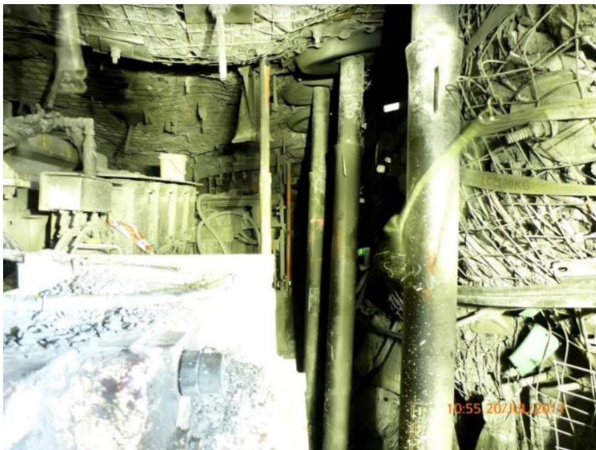
Figure 2. Impeded access due to temporary support
