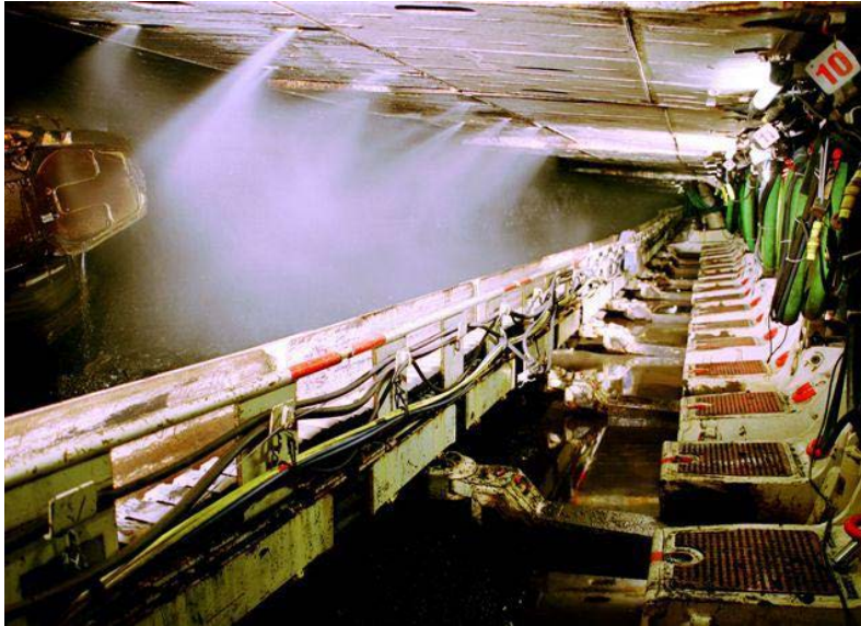
Figure 6: Shield canopy sprays
