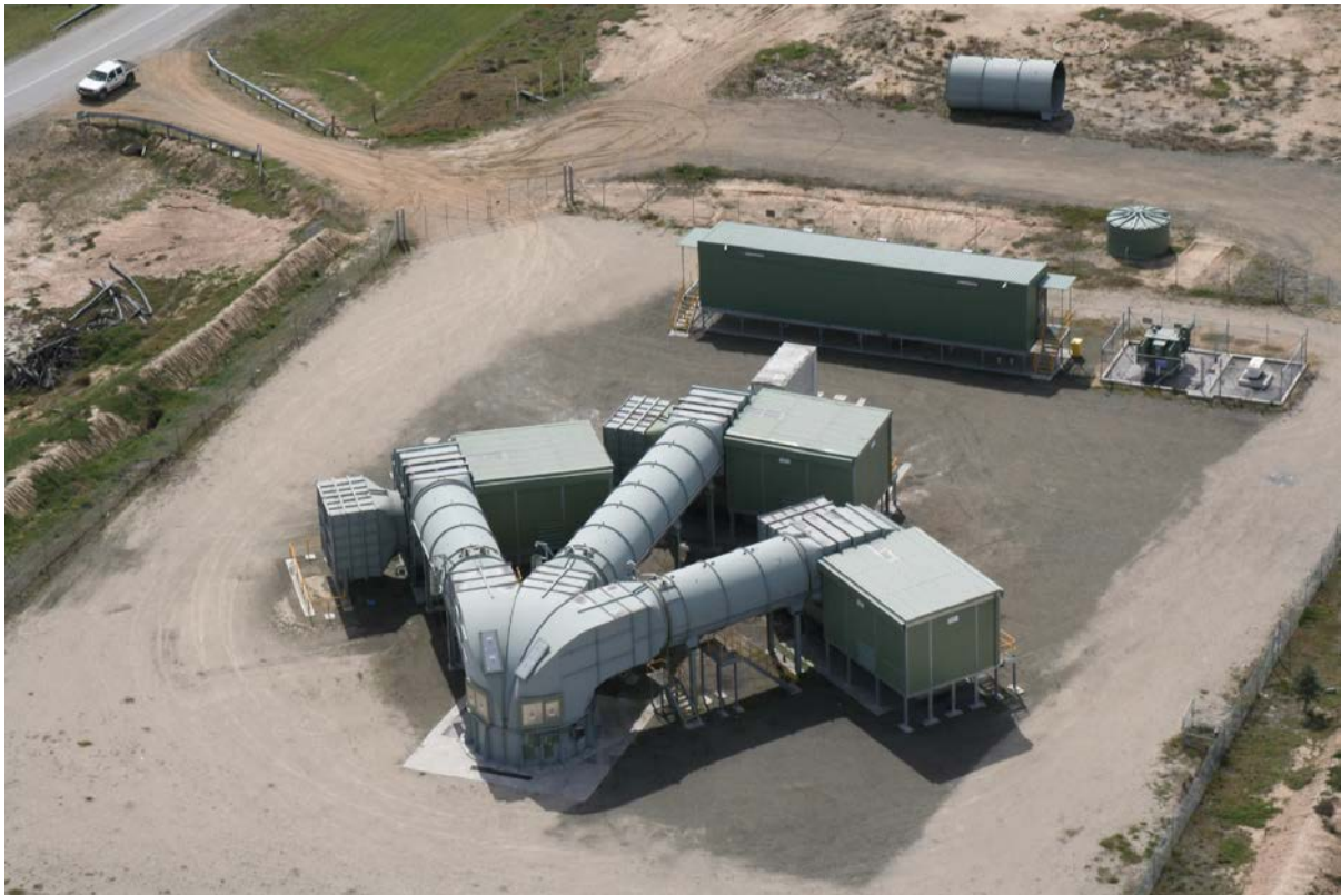
Figure 5: No 1 shaft fan installation 9
