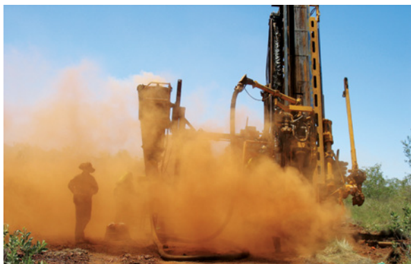
RC dry drilling
