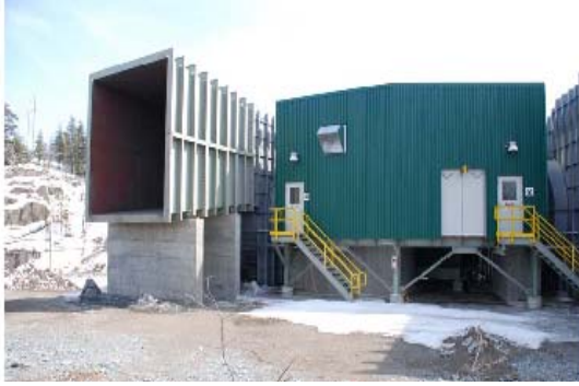
Figure 11. Vale Inco Coleman #2 Shaft Motor House
