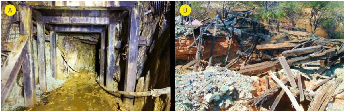
Abandoned mine workings, showing underground tunnel (A) and vertical shaft opening (B).
