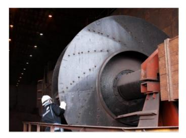
Variable speed drives were fitted to Waste Gas Sinter Fans in a steelworks and the operating regime changed. Instead of running at constant speed these fans were now running with several speed changes per day.
