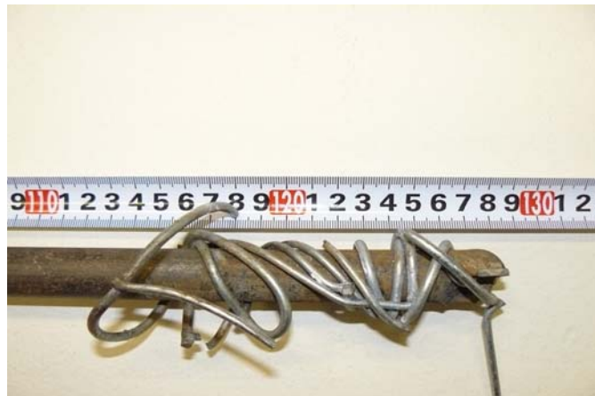
The drill steel, drill bit and entangled rib mesh
